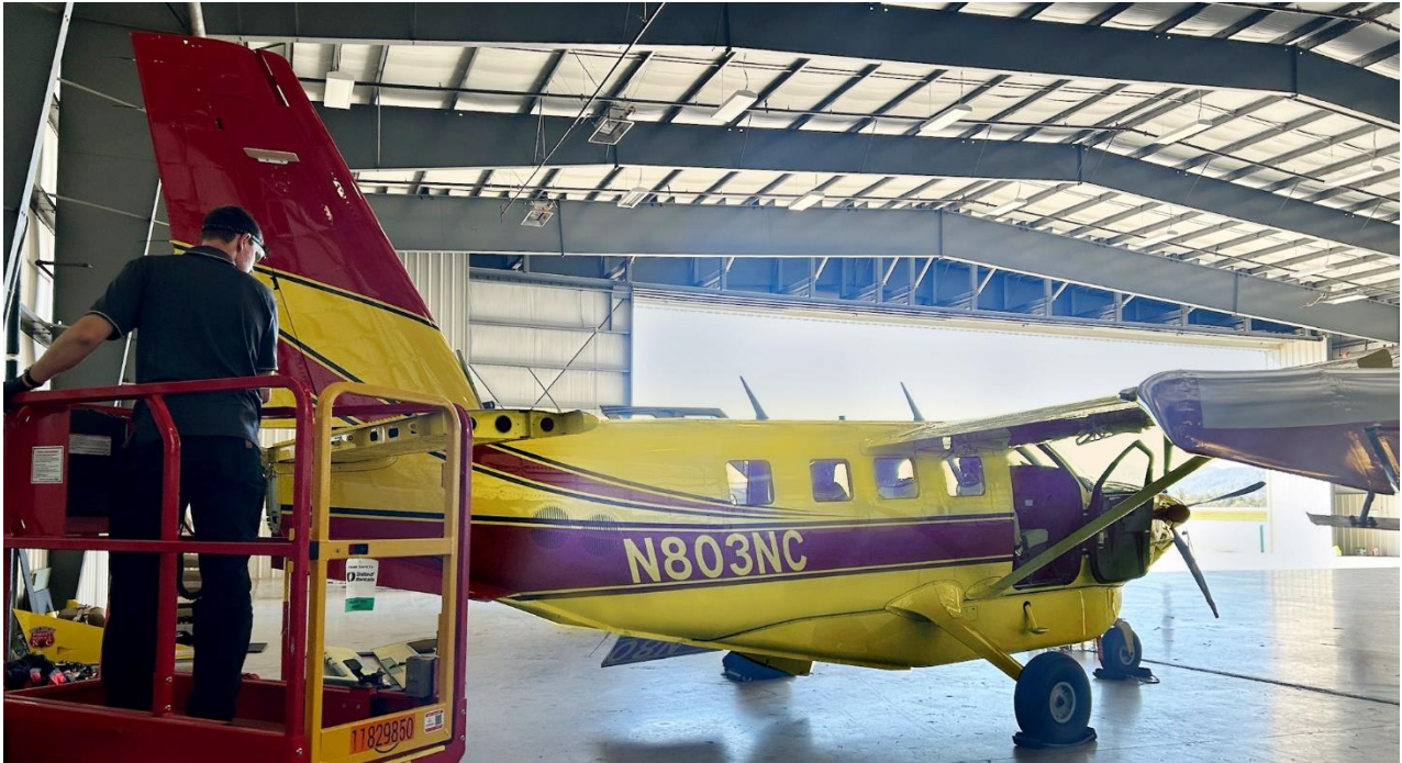
The Kodiak 100 operated by North Carolina Forest Service's Aviation Division undergoes the replacement of its elevators and repair of the rudder by Daher's Kodiak Care team at Asheville Regional Airport.
